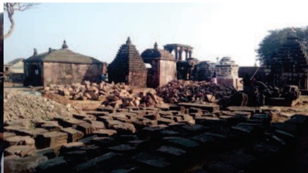
Fig.3 ongoing work of ASI (Source: Author) with the students. (Source: Author)
